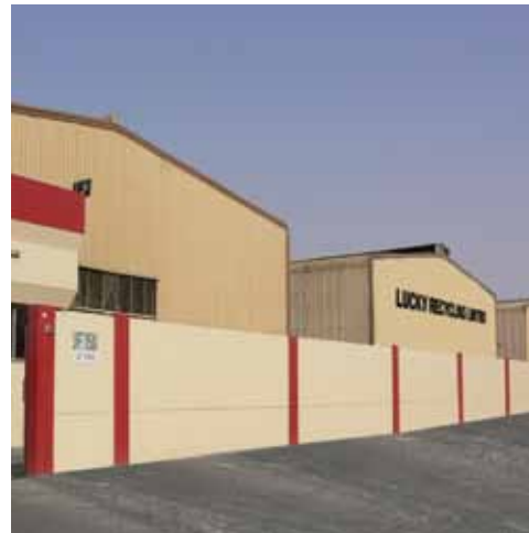
The Lucky Group's recycling facility in Jebel Ali Free Zone - Dubai, United Arab Emirates
